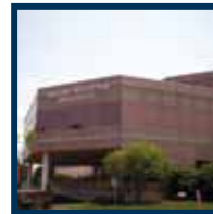
Cleveland East, Ohio
